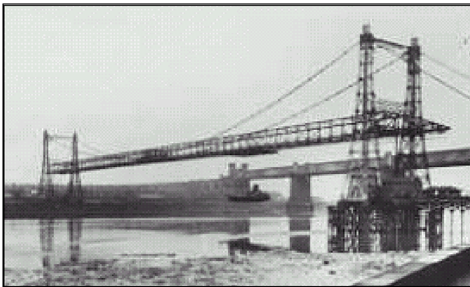
The Runcorn Transporter Bridge with the Old Bridge in the background
